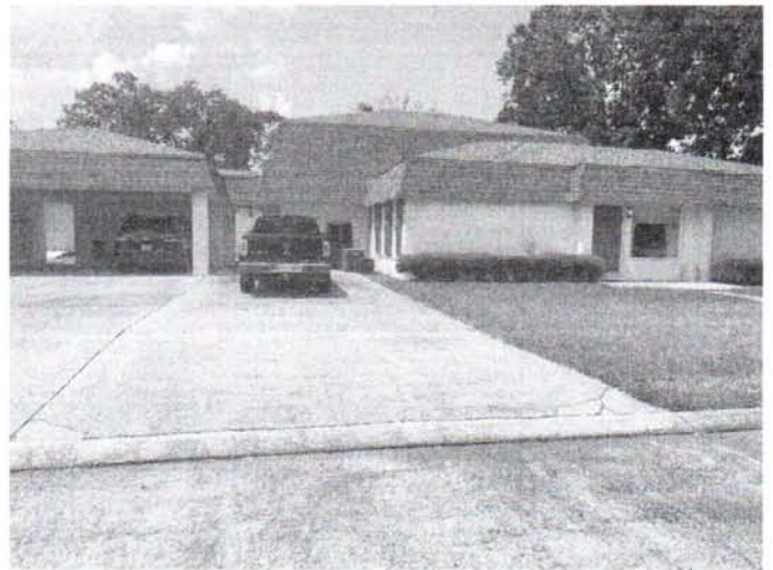
View of office entrance and parking available. The driveway can fit 6 vehicles.
