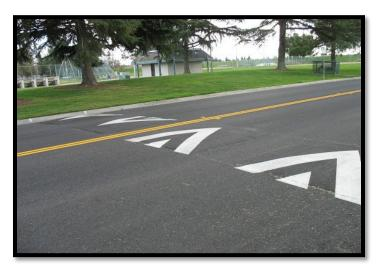
Speed humps are raised curved traffic calming devices that are 12 feet long, and 3 to four inches high. They reduce traffic by 40-60% and reduce the number of collisions on a street. Speed humps are the preferred alternative to speed bumps since they are less likely to damage vehicles or contribute to road departures due to their size and shape.
