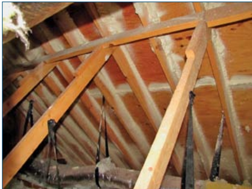
FIGURE 4-9: Example of SPF adhesive application to secure roof deck panels
