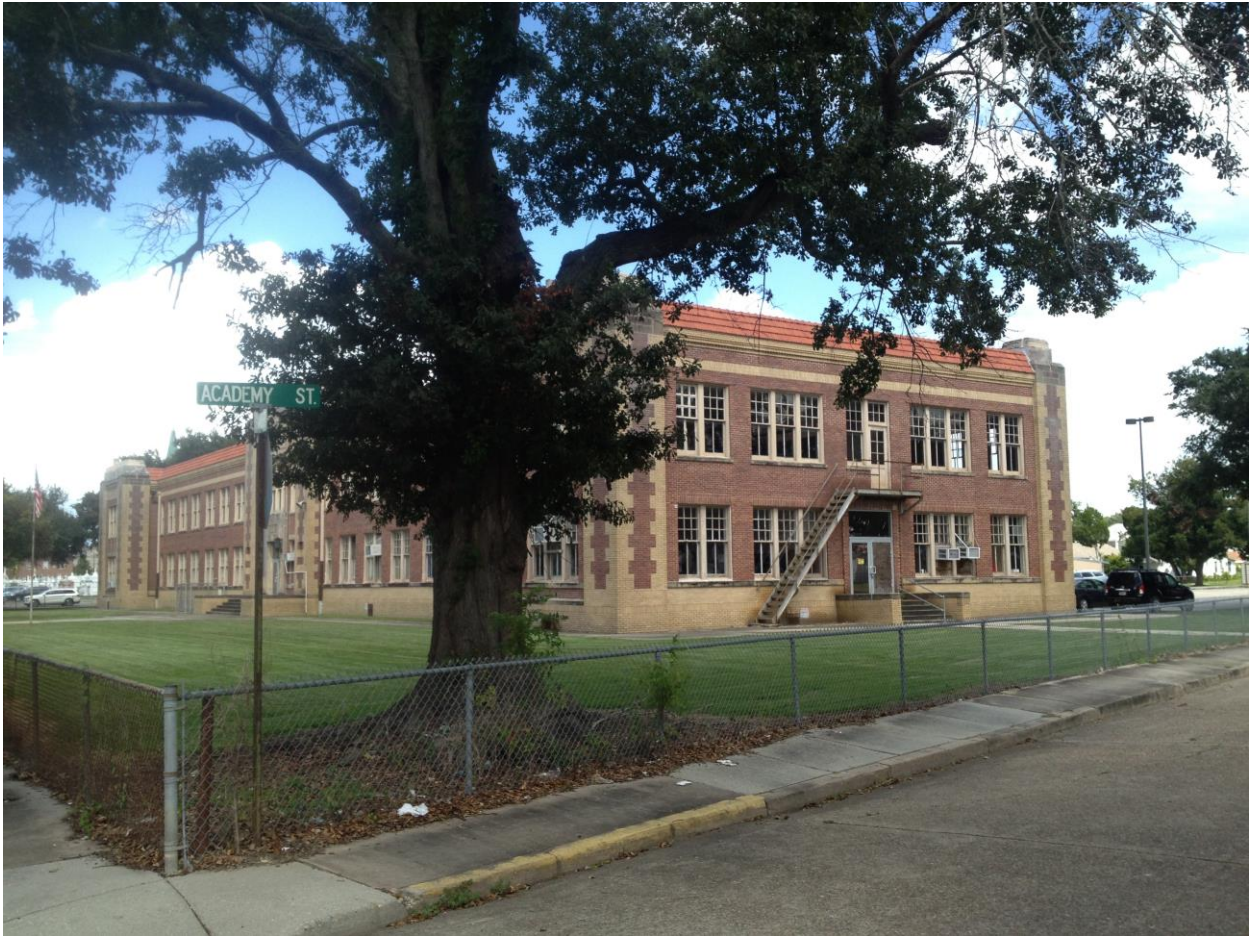
Additional front view of subject property
