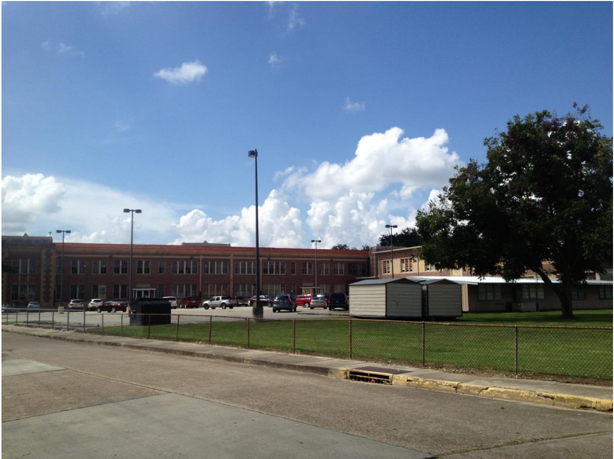
Front view of subject property from Academy Street
