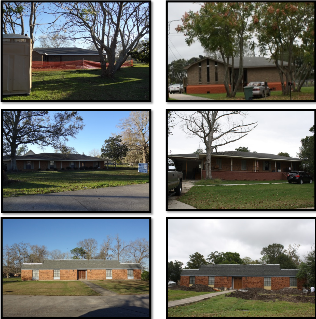
Figure 6 - Elevated Homes in Roberta Grove
