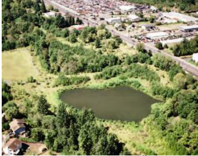
Figure 10 - Retention Pond, Source: EPA 25
